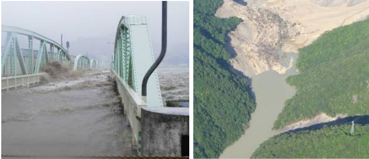
Figure 2. Effects of STS Talas (1112). Left: the Kumano River flowing over Kumano Bridge (photo: Kinan Office of River and National Highway). Right: landslide-dammed lake in Nara Prefecture (photo: JMA)
